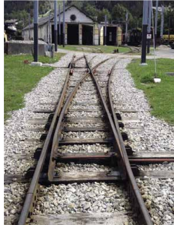
Aiguillages - écartement = 1000 mm Switches - gauge = 1000 mm
