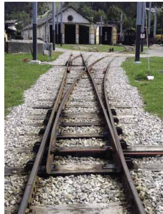
Aiguillages - écartement = 1000 mm Switches - gauge = 1000 mm
