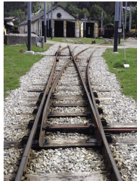
Aiguillages - écartement = 1000 mm Switches - gauge = 1000 mm
